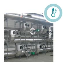
HVAC & Swimming Pools A light-weight body, a thin disc and the possibility of mounting various actuators make Aquaria plus the ideal valve for HVAC & Swimming Pool applications.
